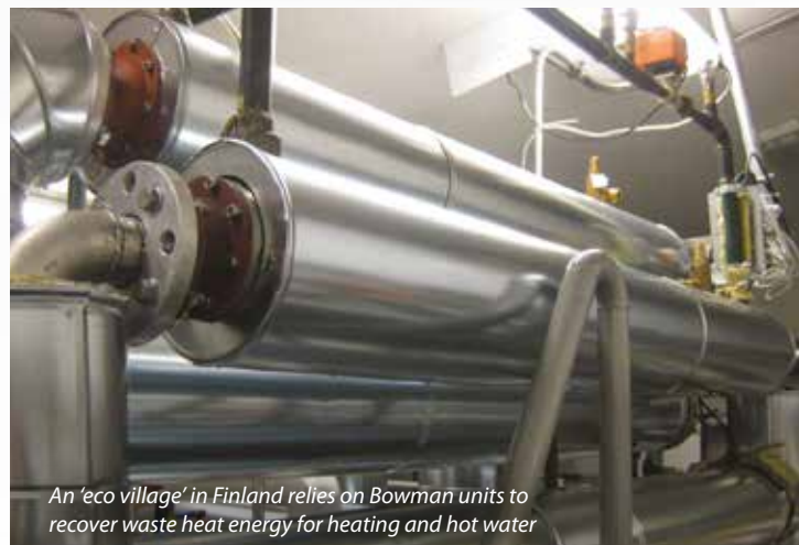
In Canada, Bowman exhaust gas units within a Cogen system, provide heat for a remote 'off-grid' community
